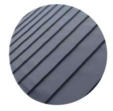
Zinc is flexible and can be used for curved roofing and cladding. It is durable, aesthetically refined, and works best when supported by a strong framework to create flowing, sculptural roof forms.
